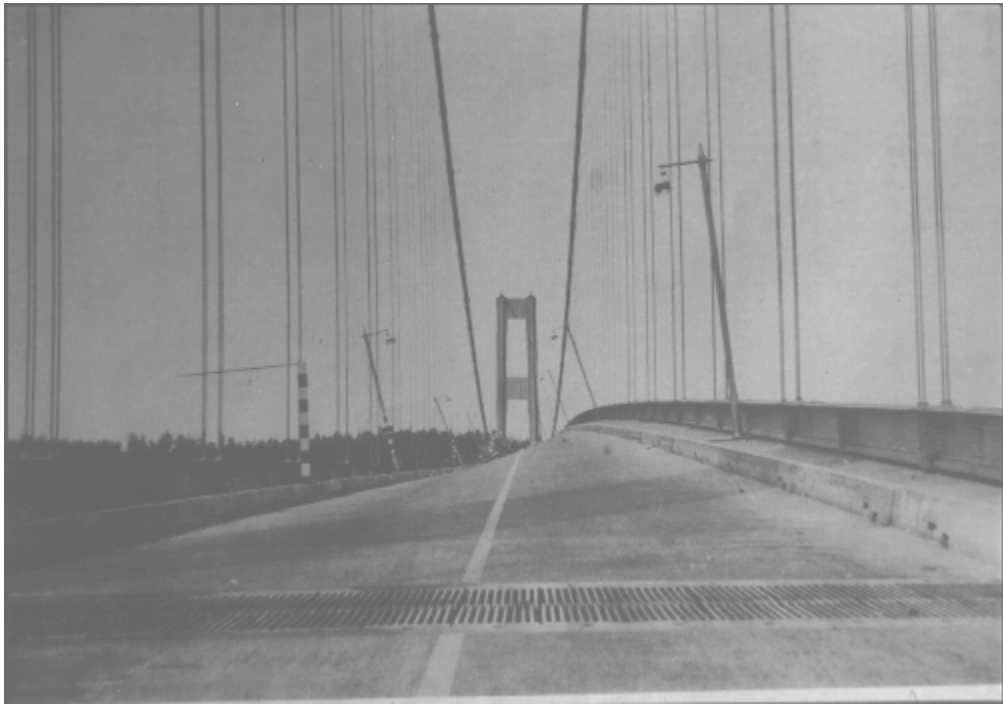
Figure 1b. Torsional Mode of the Tacoma Narrows Bridge
