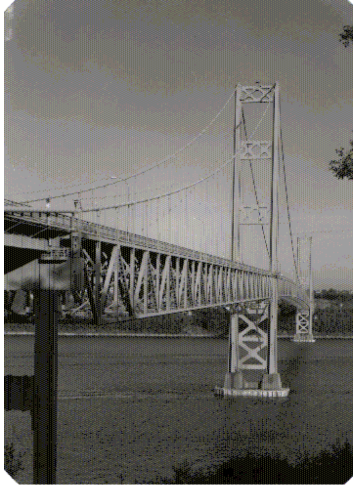
Figure 5. The Replacement Tacoma Narrows Bridge, Built in 1950
