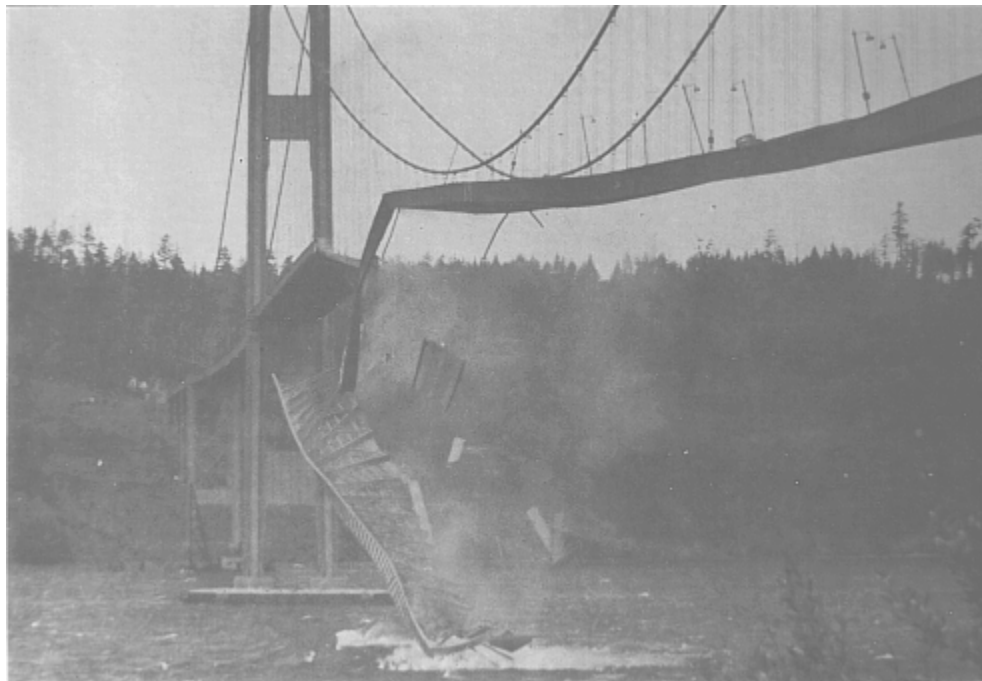
Figure 2a. Failure of the Tacoma Narrows Bridge
