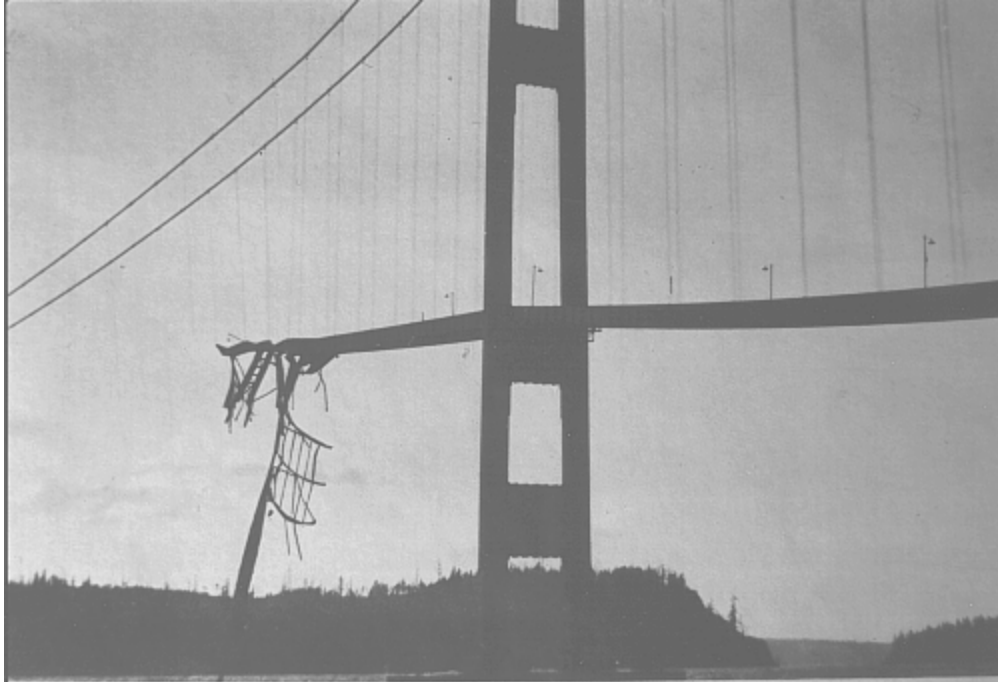
Figure 2b. Tacoma Narrows Bridge after the Failure
