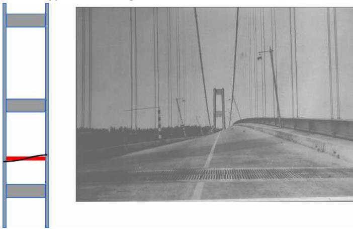
**The failure of the bridge occurred when a new type of twisting occurred. This twisting, rather than longitudinal was torsional.**
